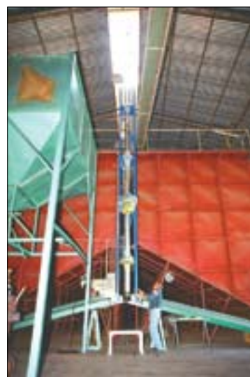
Installation of an Olds Elevator.
