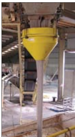
The Dust Suppression Hopper in action.
