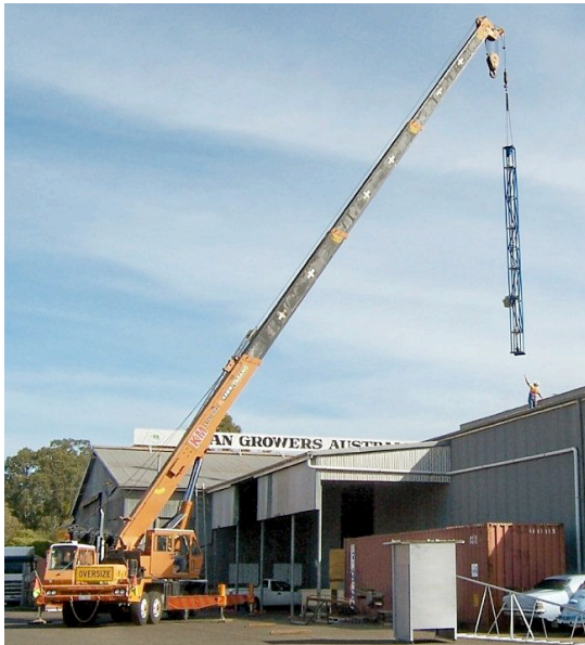
Figure 15 – 152 mm (6") by 10.7 metres lift Olds Elevator is lowered into position at Bean Growers Australia, Kingaroy plant April 2006.
